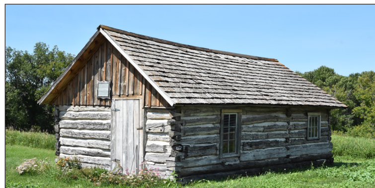
The Bernard Bernhardson House in Comstock, Minnesota, built in the 1870s by the first-known Swedish settler family along the Red River of the North. The home is on the National Register of Historic Places. USACE photo by Patrick Moes
